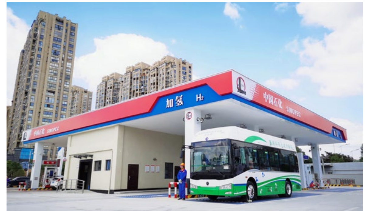
Hydrogen refuel station in Jiaxing, Zhejiang
