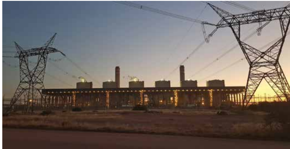
Five units at Medupi Power Station have been synchronised to the grid, denoted by the lights on top of the boiler housing.
