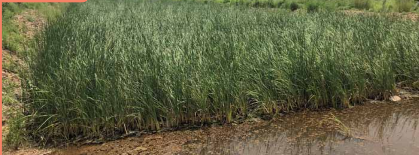
Constructed wetlands at Loulo, Mali.
