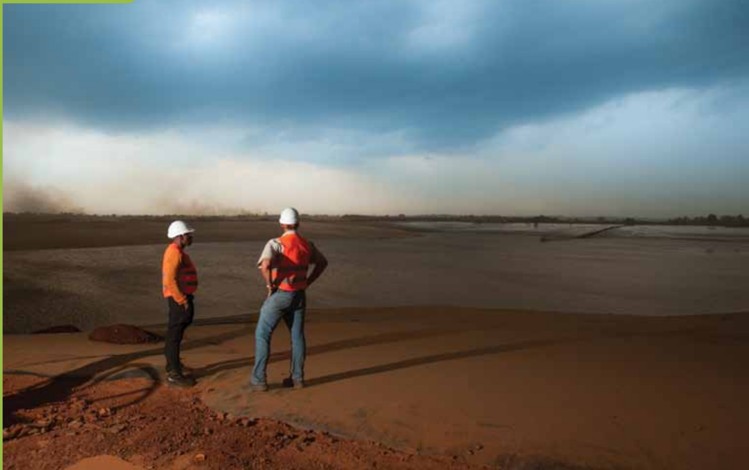
Tailings dam at Loulo, Mali.
