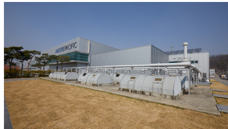
Expansion of the rainwater storage facilities
