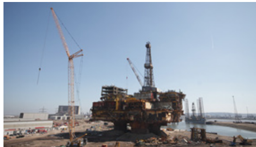
In 2018, we made significant progress in dismantling the topside.
