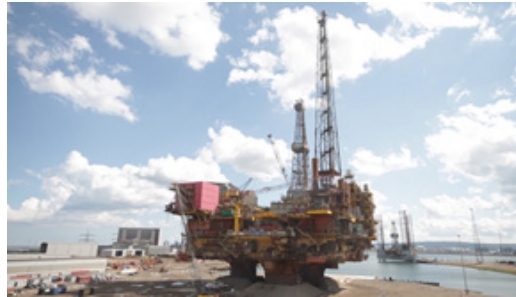
The 24,200-tonne Brent Delta topside, which was removed and brought onshore in 2017, is being recycled in Hartlepool, UK.
