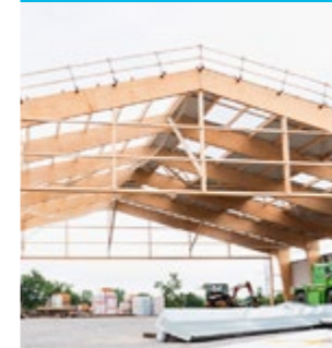
Building components and systems
