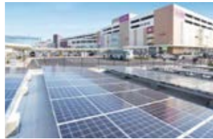
Solar panel installation
