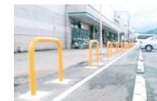
Parking lot guardrails
