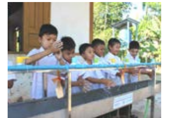
Children washing their hands at new water supply facilities (Myanmar)
