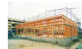
A store under construction (Ministop Co., Ltd.)
