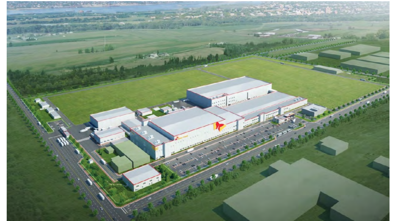
Establishing battery production facilities in Hungary (Expected to be completed by 2020)
