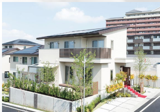
Energy self-sufficient housing (SECUREA Toyota Kakimoto)
