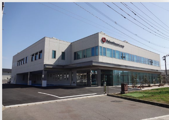
Electricity self-sufficient building (Daiwa House Saga Building)
