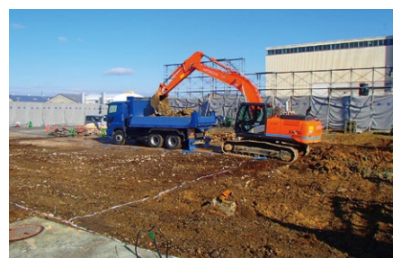
Loading work of contaminated soil in Nara Plant
