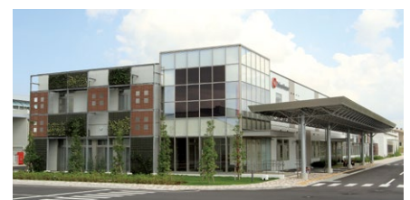
Daiwa KOMFORT (our Ryugasaki Plant Office Building)
