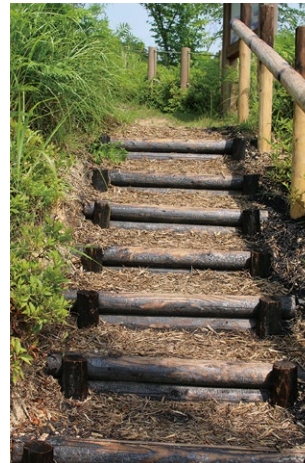
Path to Taikohanamizuka repaired and improved in Fiscal 2017
