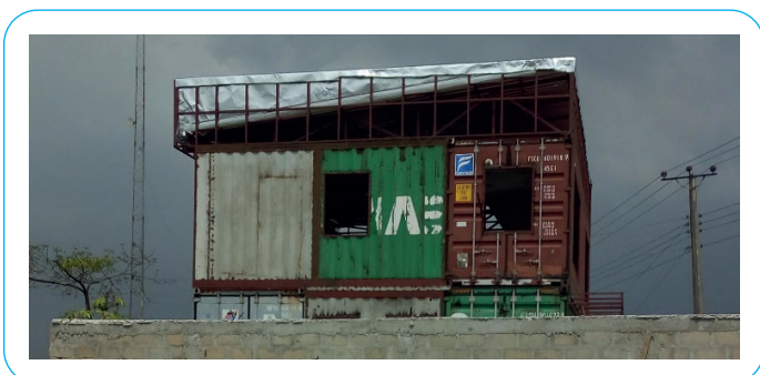
QIT Branch (Construction in progress)
