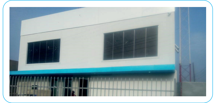
QIT Branch (Completed)
