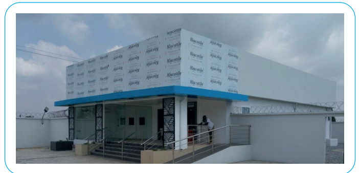
LASU Branch (Completed)
