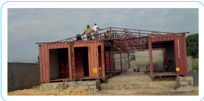
LASU Branch (Construction in progress)
