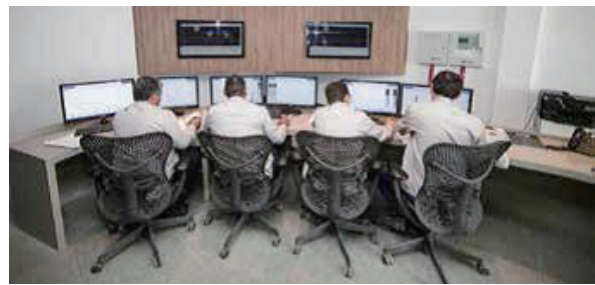
Central control room
