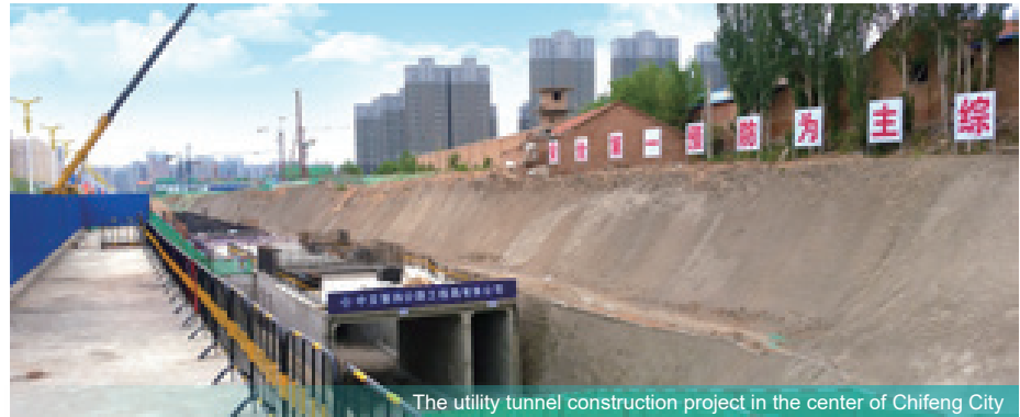
The utility tunnel construction project in the center of Chifeng City
