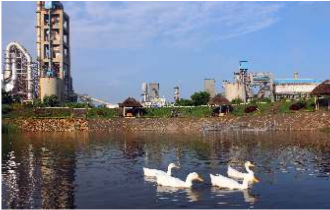
Rain fed artificial lake created at the Ariyalur Plant in Tamil Nadu.
