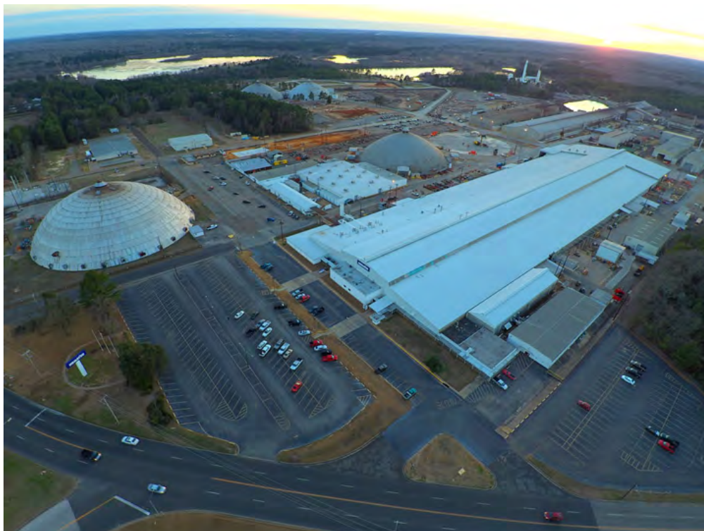
KMC Longview, TX Facility
