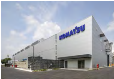
New heat treatment plant
