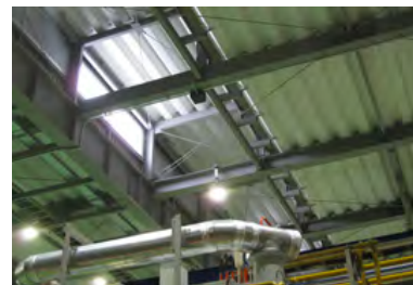
Natural evocation utilizing lighting due to indirect nature maximum and negative pressure generated in indentations of the roof
