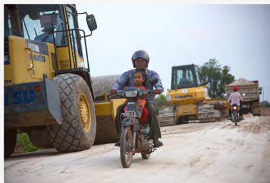
Road construction using Komatsu equipment
