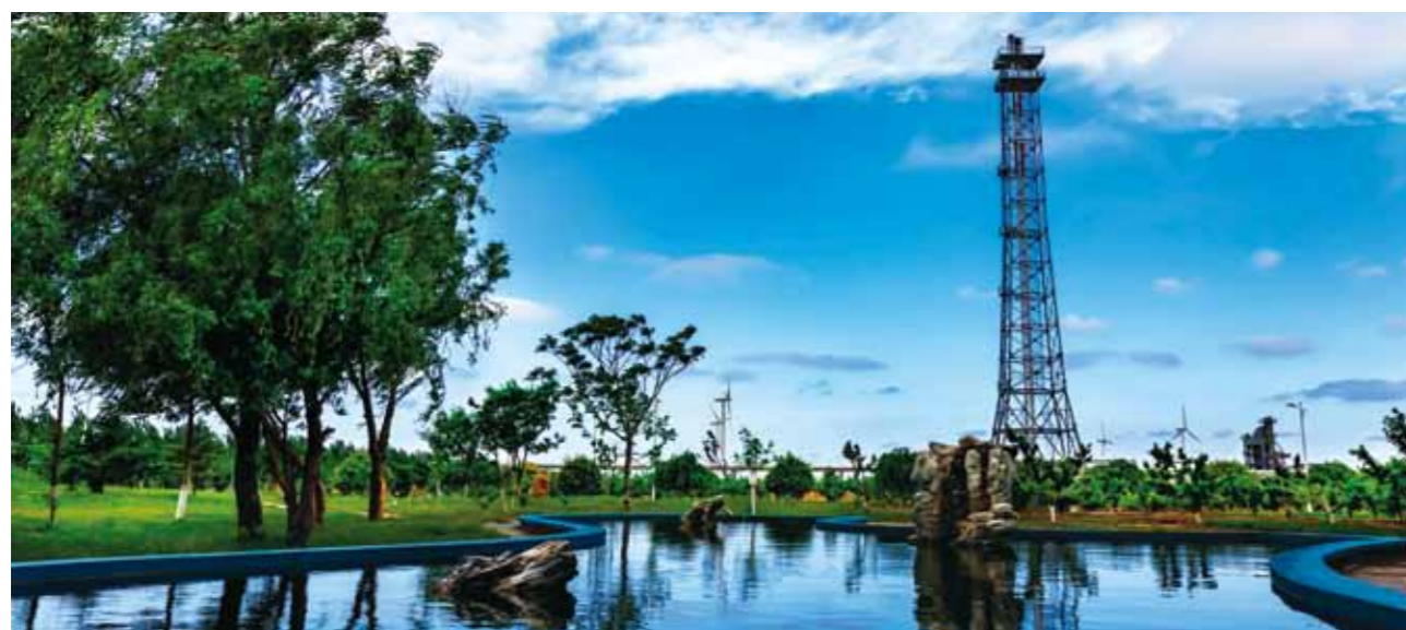
Yingkou Natural Gas Processing Plant
