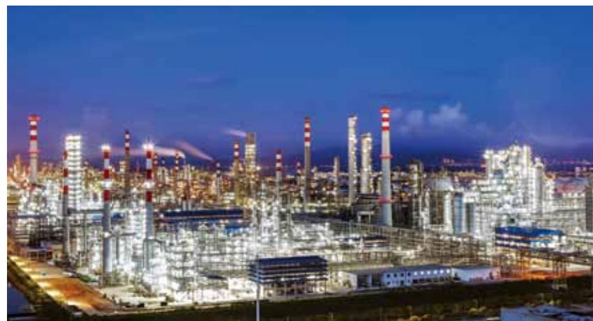
Night scene of the project site of Huizhou Refinery Phase II
