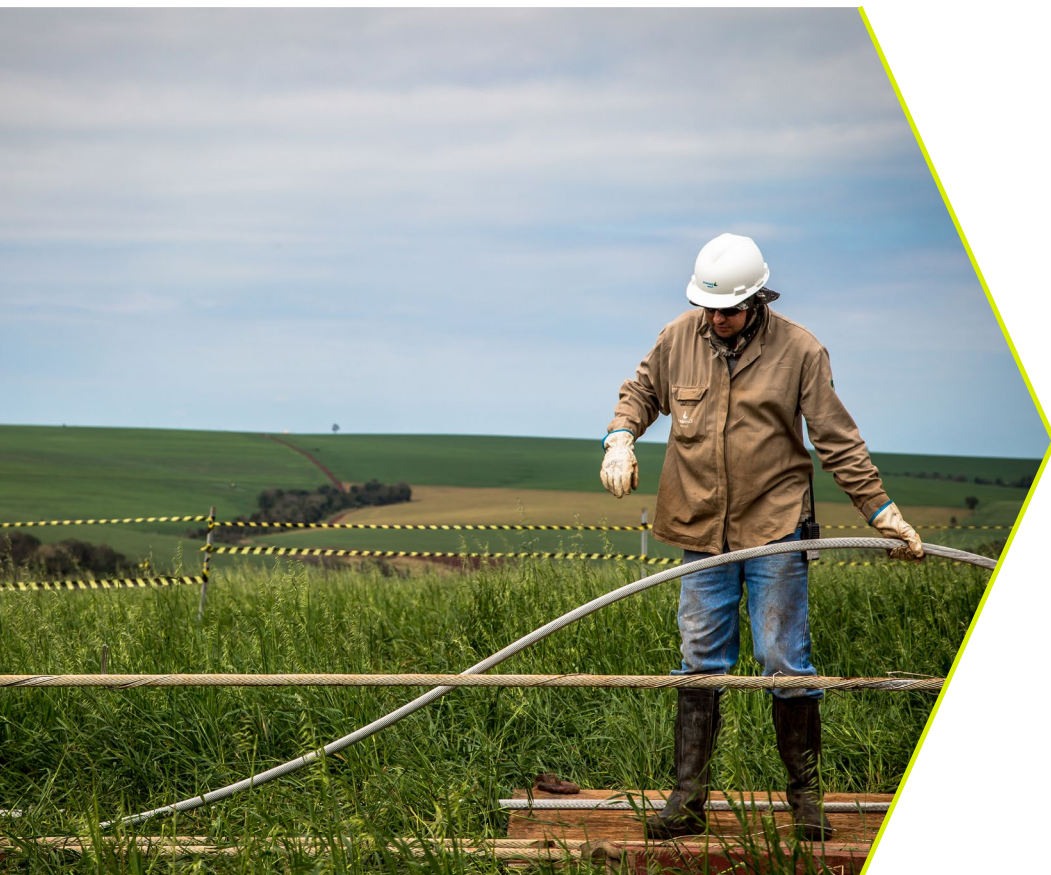
Repair work at TL – Eletrobras Furnas/Daniela Monteiro
