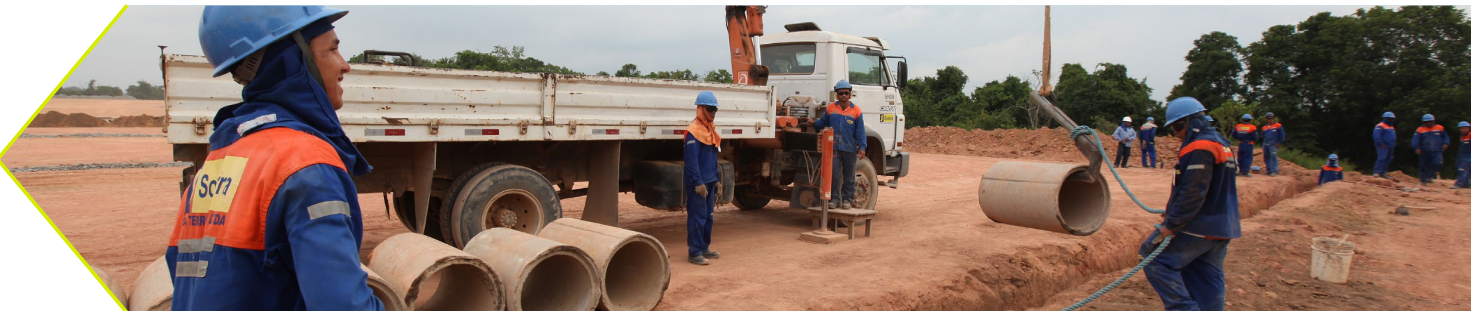
TL Construction Tucuruí-Manaus - Eletrobras holding / Jorge Coelho
