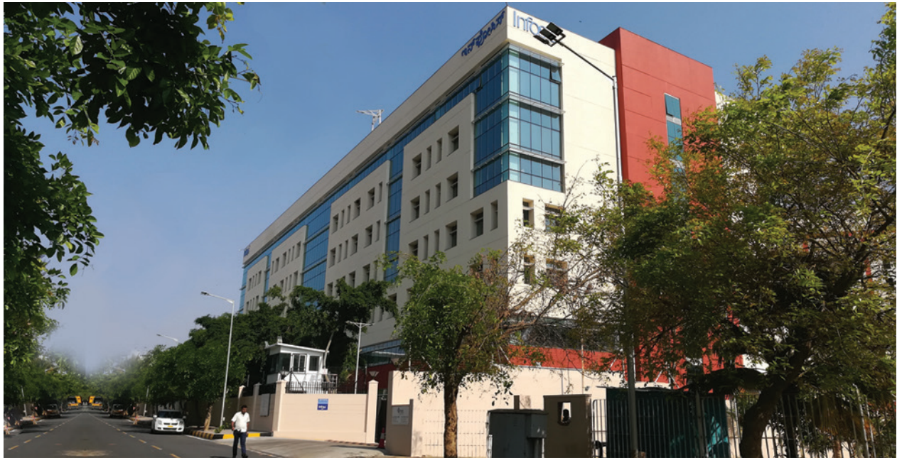
EC 40, Bengaluru is a fully prefabricated building commissioned in 2017
