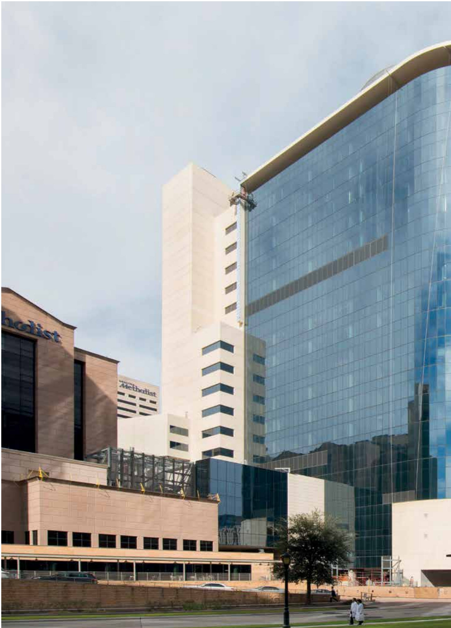
Work constructed with Argos ® products: Methodist Hospital in Houston, Texas, United States.
