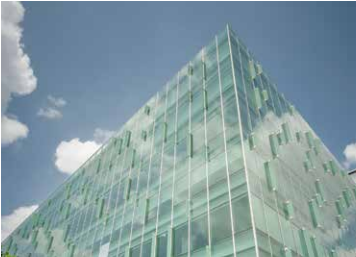
Sustainable Construction: Panama Administrative Office, Caribbean and Central America Region
