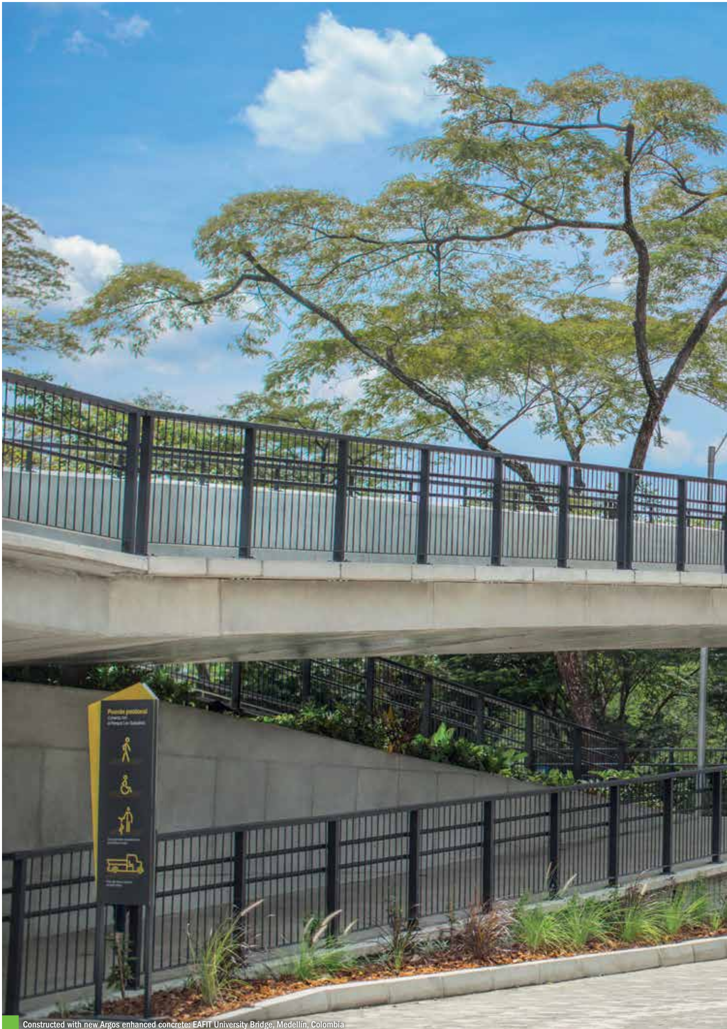
Constructed with new Argos enhanced concrete: EAFIT University Bridge, Medellín, Colombia
