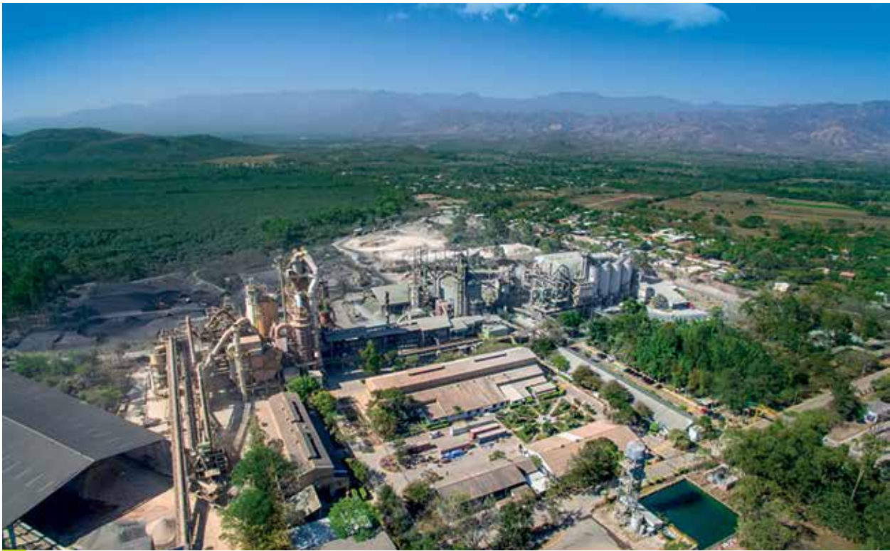
Comayagua Plant, Honduras, Caribbean and Central America
