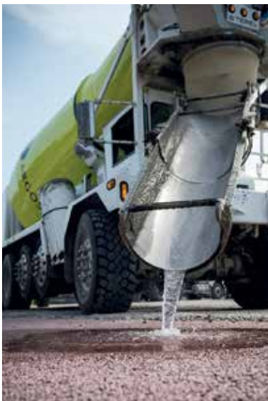
Permeable Concrete, United States
