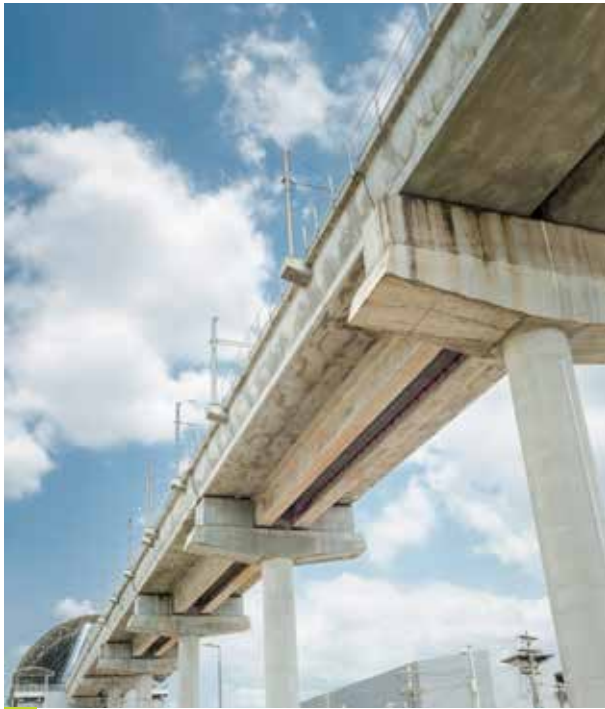
Infrastructure project built with Argos: second line of the Metro of Panama
