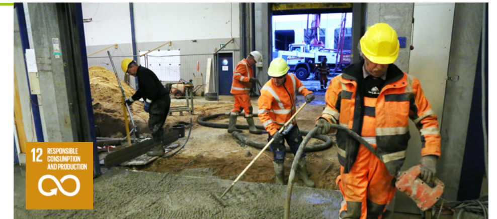
We completed decontamination in October 2017
