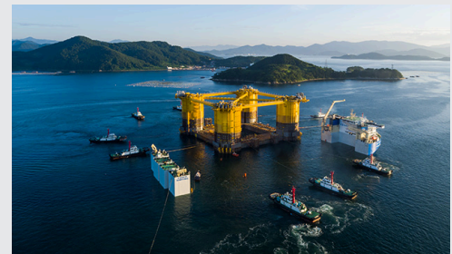
The Appomattox project hull is prepared for its journey from Geogje, South Korea to Ingleside, Texas, USA, to complete the semi-submersible host platform's construction.
