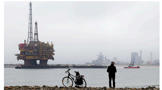
The Brent Delta platform was transported to the Able UK Seaton Port yard in Hartlepool, UK, where at least 97% of the material will be recycled.
