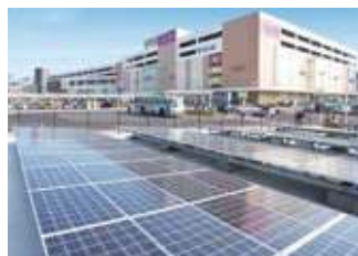
Solar panel installation
