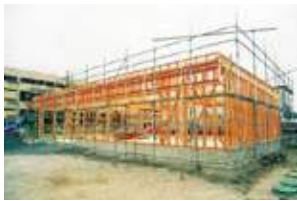
Store under construction
