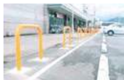
Parking Lot Guardrails
