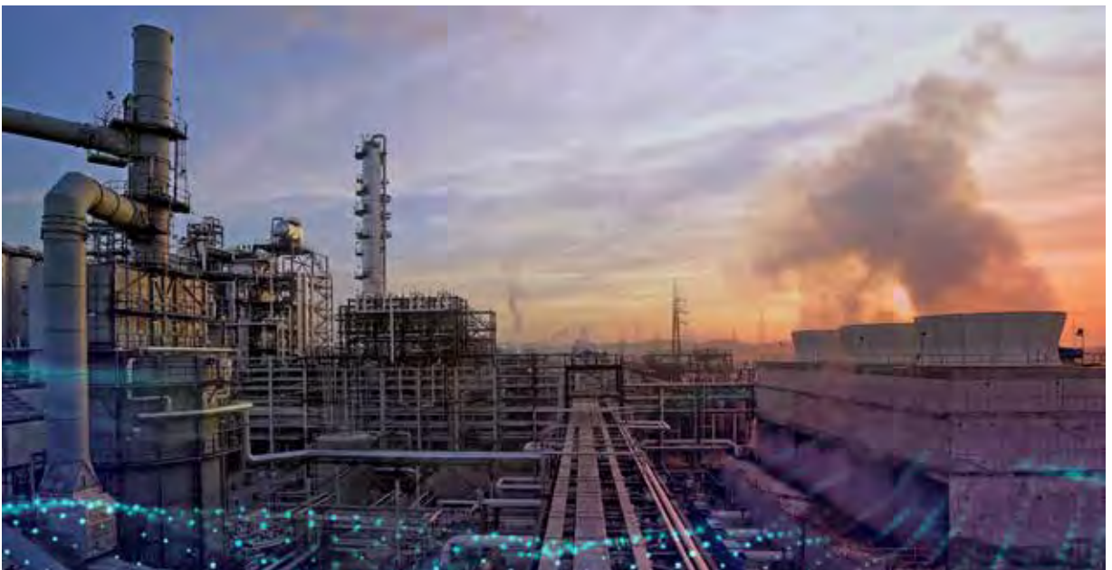
Front view of SSNC(SABIC SK Nexlene Company) Ulsan Plant
