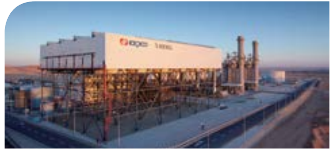
Power plant in Al-Qatrana, Jordan
