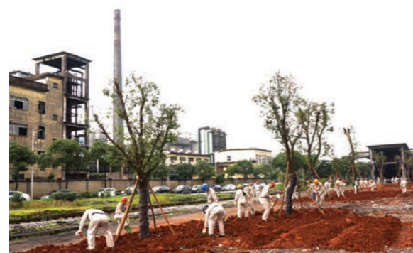
Landscaping the old blast furnace removal area by Shaoguan Iron & Steel
