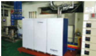
Fuel cells for Jisan Welfare Center
