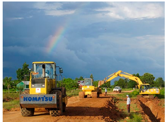
Komatsu's construction machinery developing infrastructures
