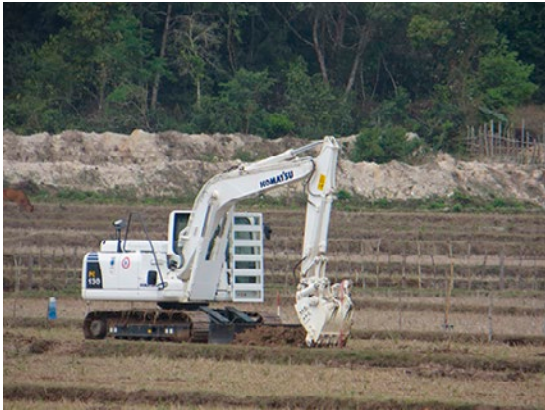
Machine developed based on a hydraulic excavator (for handling unexploded bombs)
