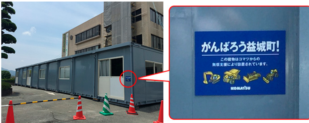
Unit houses set up in the Town Hall's parking space / A message from KOMATSU posted beside the entrance door
