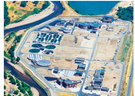
Northern Treatment Plant
