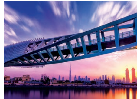
Dubai Water Canal pedestrian bridge
