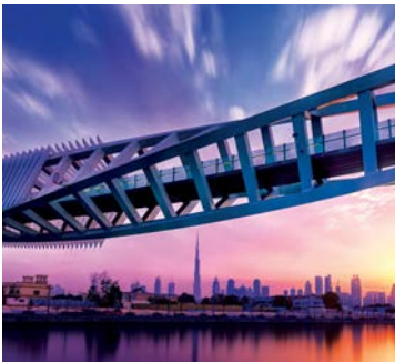
Dubai Water Canal pedestrian bridge
