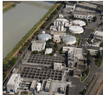
Tacoma Central Wastewater Treatment Plant
