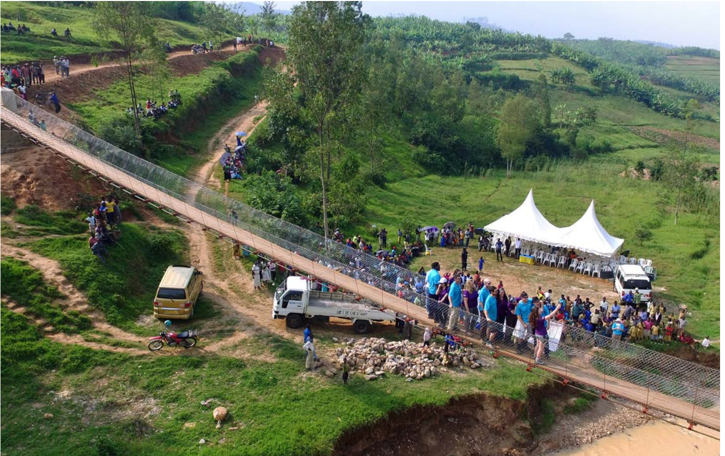
2016 Rwanda completed bridge build
