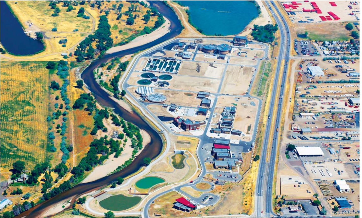
Northern Treatment Plant, Brighton, Colorado
