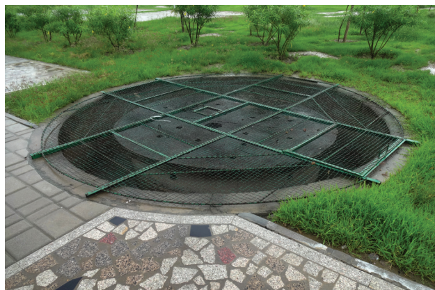
Rainwater harvesting pit at our Jaipur campus
