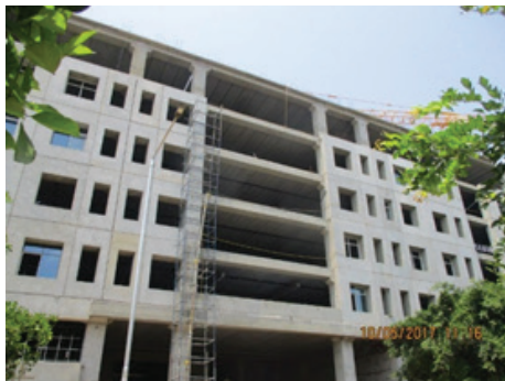
Precast construction in Bengaluru
