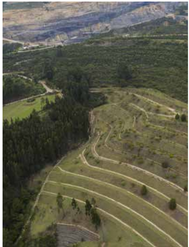
Quarry rehabilitation at Sogamoso Plant, Colombia Region
