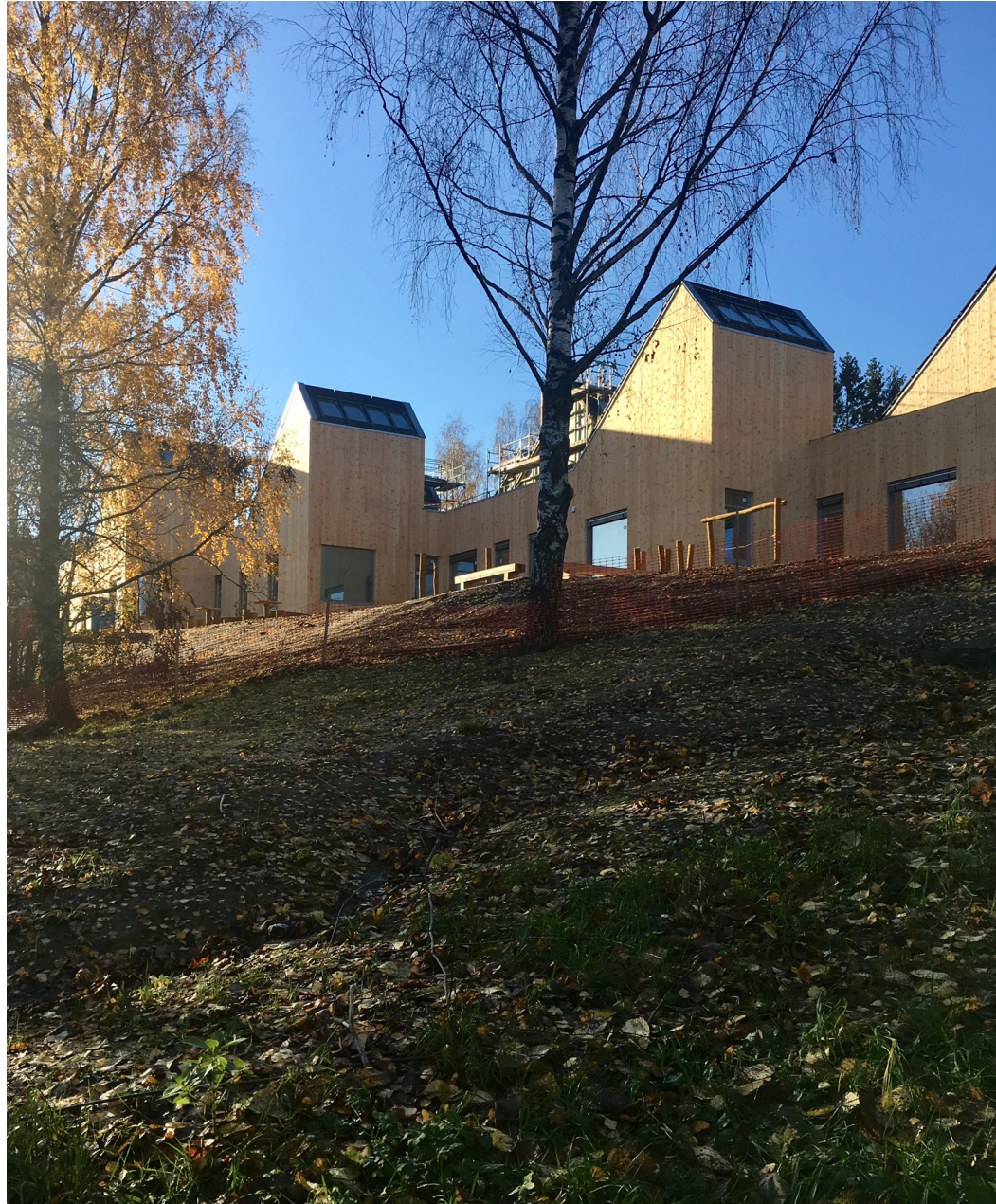
The energy-plus kindergarten Kistefosdammen, sits on a slated piece of land, providing the children with plenty of outdoor roaming space
