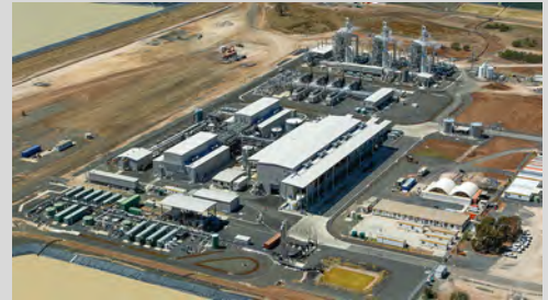
At the QGC Project, Australia, the central water treatment plant recycles salty underground water extracted during gas production.
