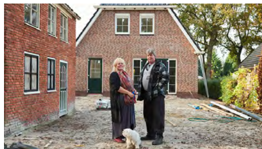
Frits and Ada Indri, who live near the Groningen gas field in the Netherlands, had their house rebuilt to be earthquake-proof after it was severely damaged due to an earthquake.
