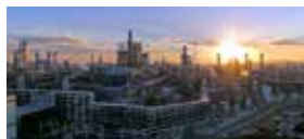
Incheon Complex PX Factory
