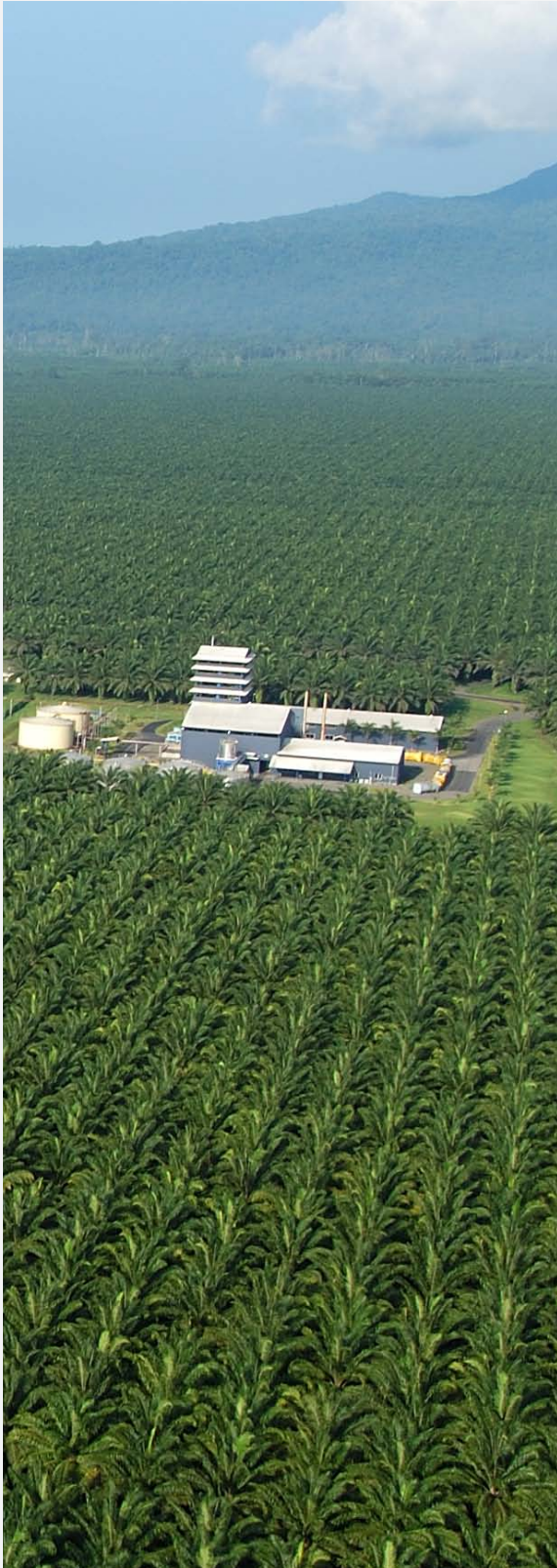
Kumbango Oil Refinery & Mill at Kimbe, West New Britain, Papua New Guinea
