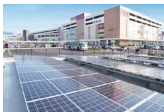
Solar panel installation
