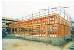
Store under construction
