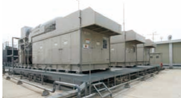
Private power generation equipment installation
