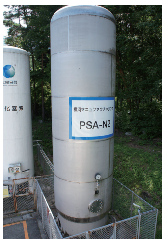
The compressed nitrogen manufacturing equipment with a PSA system
