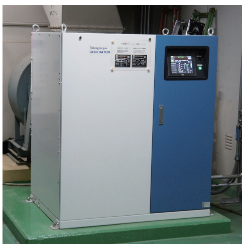
The compressed nitrogen manufacturing equipment with a PSA system
