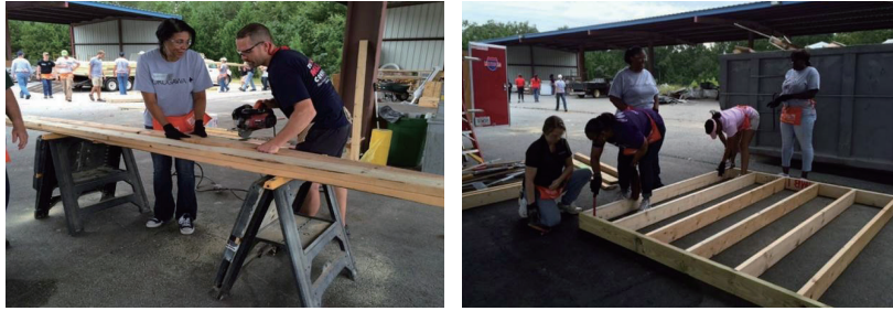
Volunteers from Yokogawa Corporation of America working at the build
