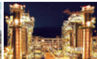
Norte II Gas-fired Combined Power Generation, Mexico
