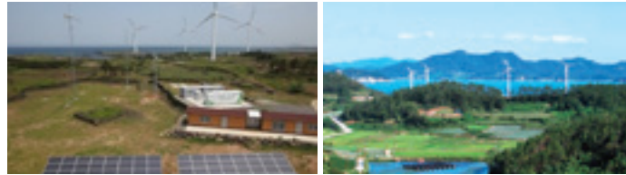
Electricity Supply to remote areas via the Micro Grid
