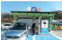
EV Charging Infrastructure
