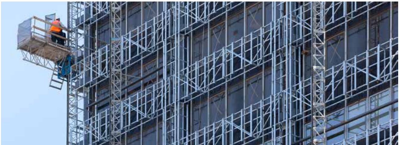
Energy rehabilitation. Málaga (Spain)
