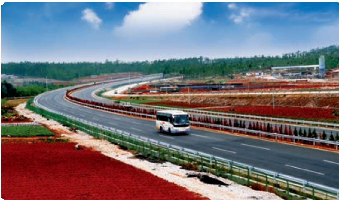
The Xishi road built with the loan provided by CDB Yunnan
