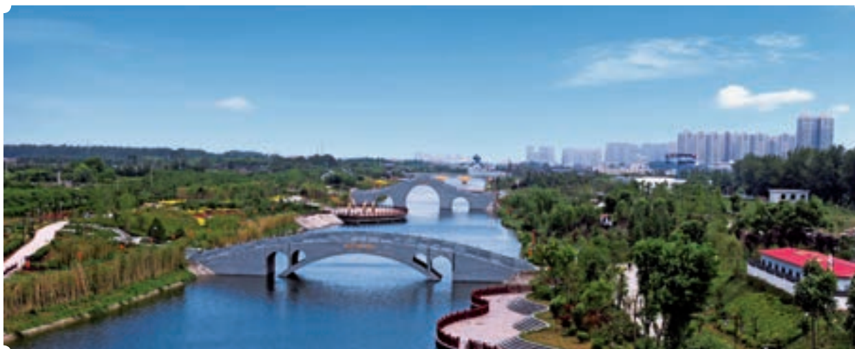
Tuanjie Serservoir control project in Xi'an financed by CDB Shaanxi. The project removed all the solid refuse hills around it and improved the surrounding environment, protected the ruins of the ancient city and raised its capacity of resisting floods.
