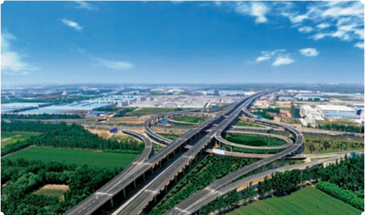
The interchange project in northern Dezhou financed by CDB Shandong. By the end of 2015, CDB Shandong had financed 20 national and provincial highways in Shandong Province, accounting for 37 percent of local expressways in service.
