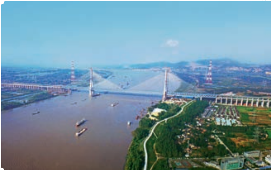
Hefei-Fuzhou Railway Yangtze River Bridge at Tingling, Anhui Province
