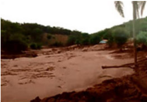
Condition of collapsed dam
