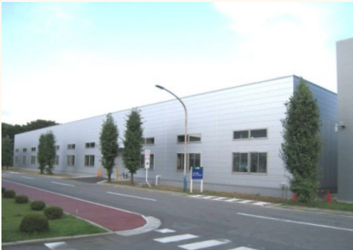
The newly completed technical training center
