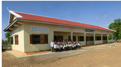
Seventh elementary school in Roung village, completed in May
