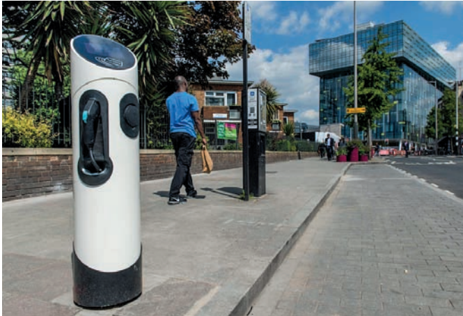
Charging terminals in London.
