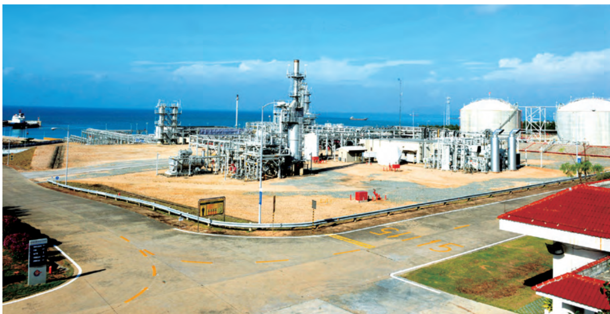
▲ Garden plant located in the Sanya City, Hainan Province—CNOOC Nanshan Terminal
