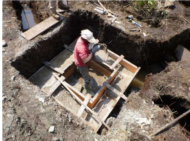
Stephen Clark, CH2M project manager, constructing a spring source collection system
