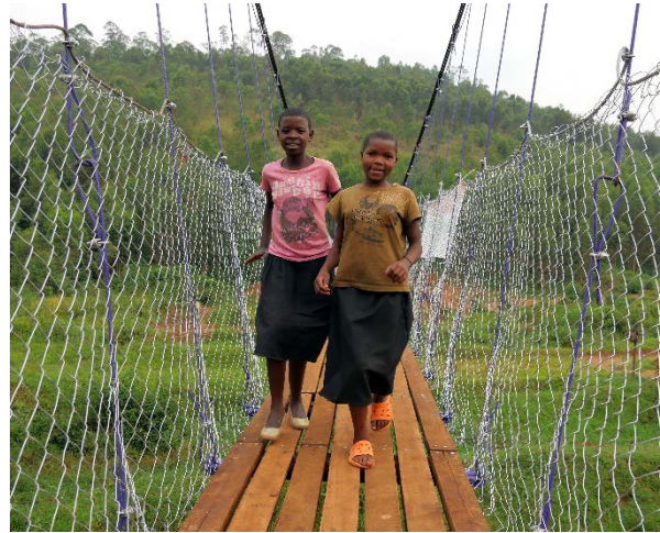
Children crossing a CH2M-constructed pedestrian suspension bridge in Rwanda
