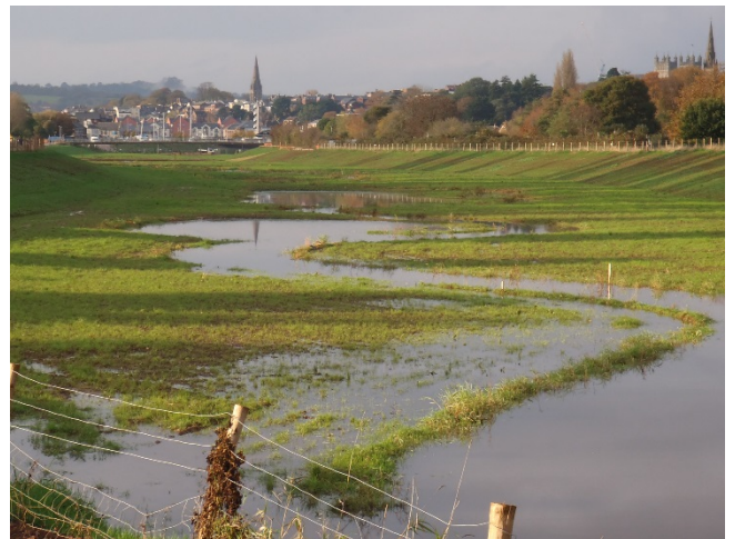
Trews flood relief channel (Exeter) incorporating wetland habitat
