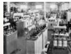
Siemens installs Brazil's first transformer plant, in São Paulo (SP).
