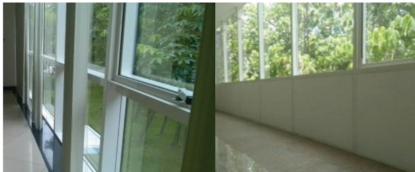
Façade retrofit: before (left) and after (right)
