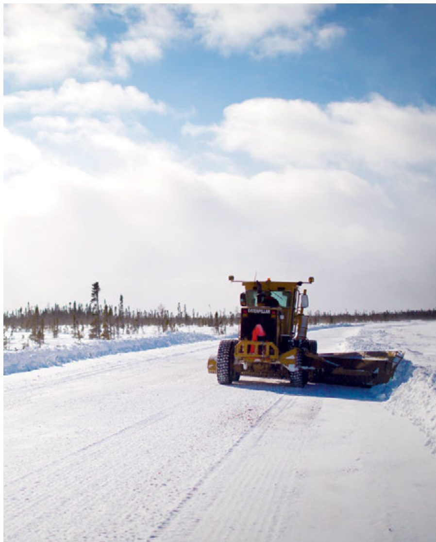
Left: Canada – Victor Mine, a logistics crew member grades the Victor Mine South Winter Ice Road.
