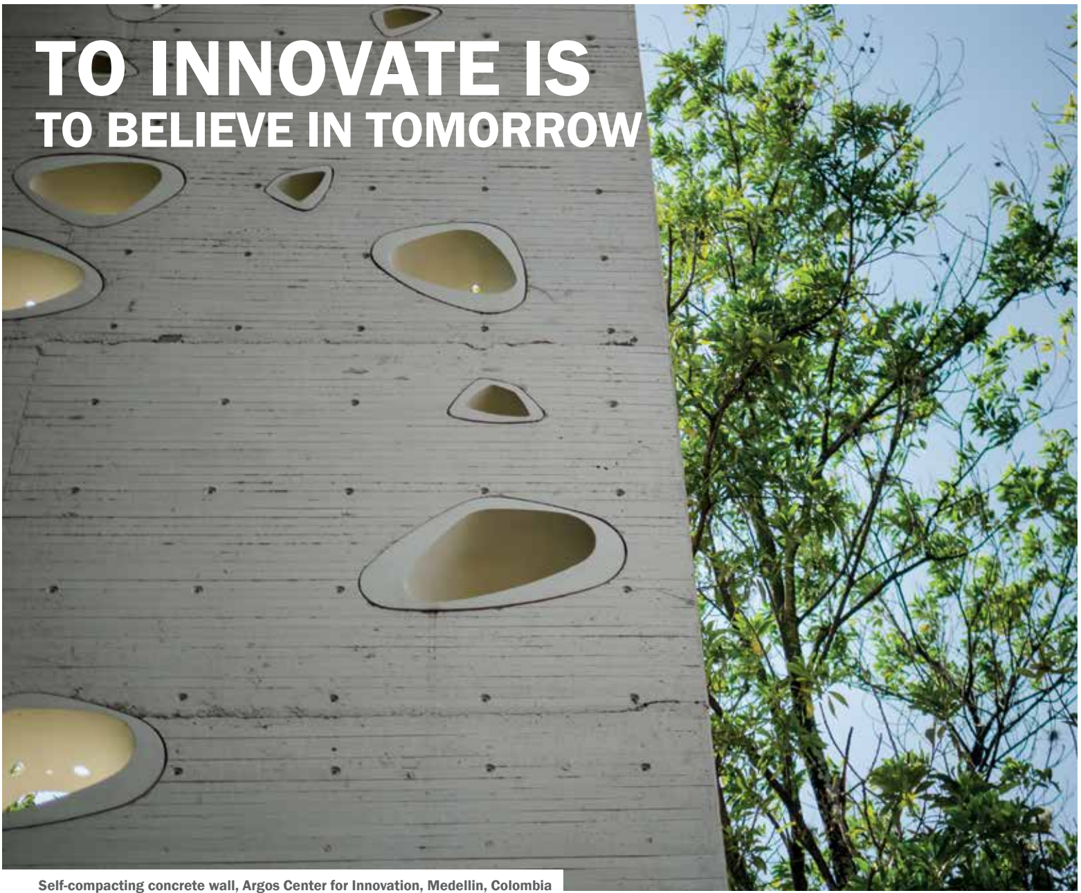
Self-compacting concrete wall, Argos Center for Innovation, Medellin, Colombia
