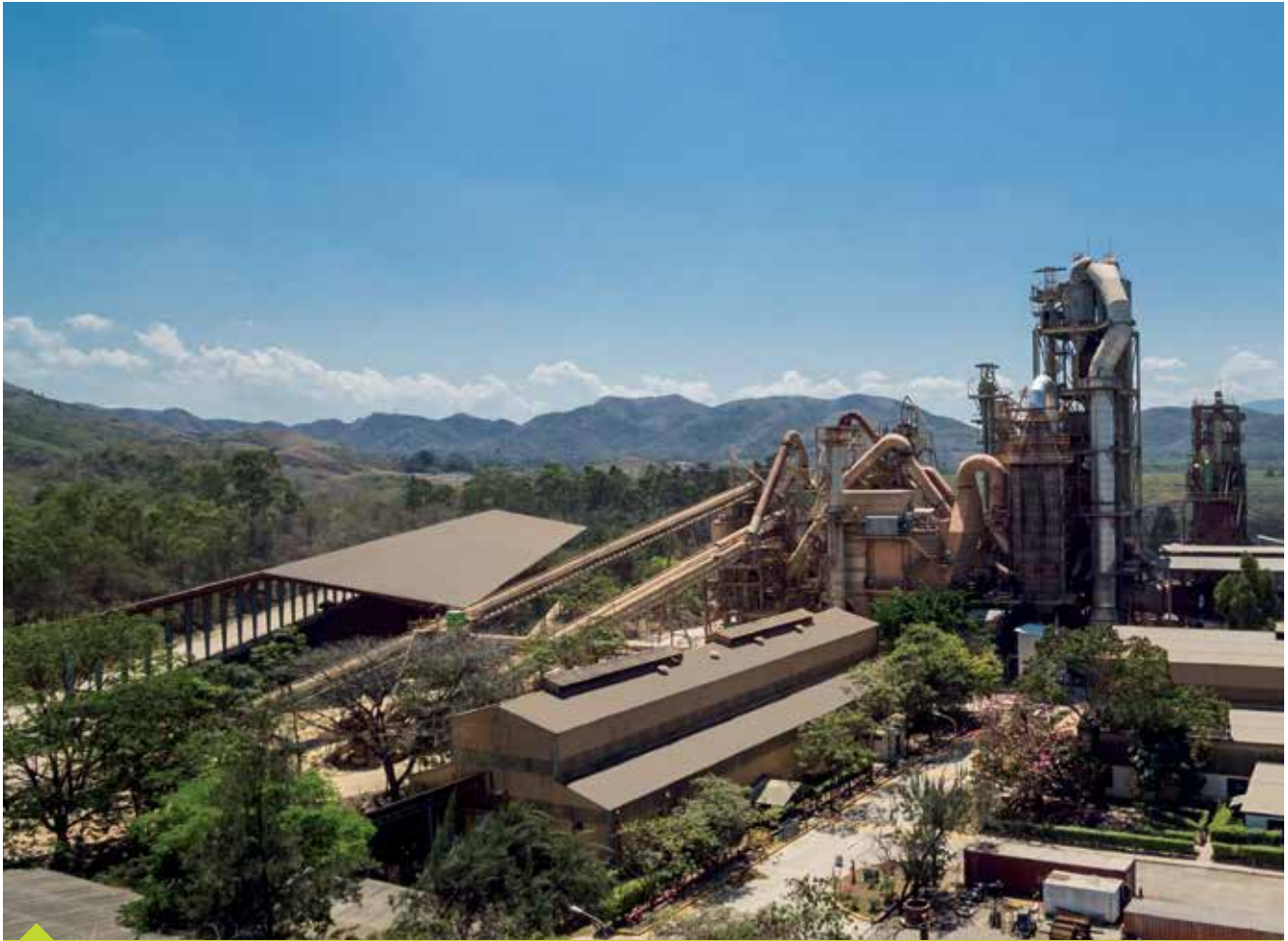
Comayagua Cement Plant, Honduras, the Caribbean and Central America Region
