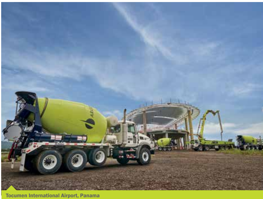
Tocumen International Airport, Panama
