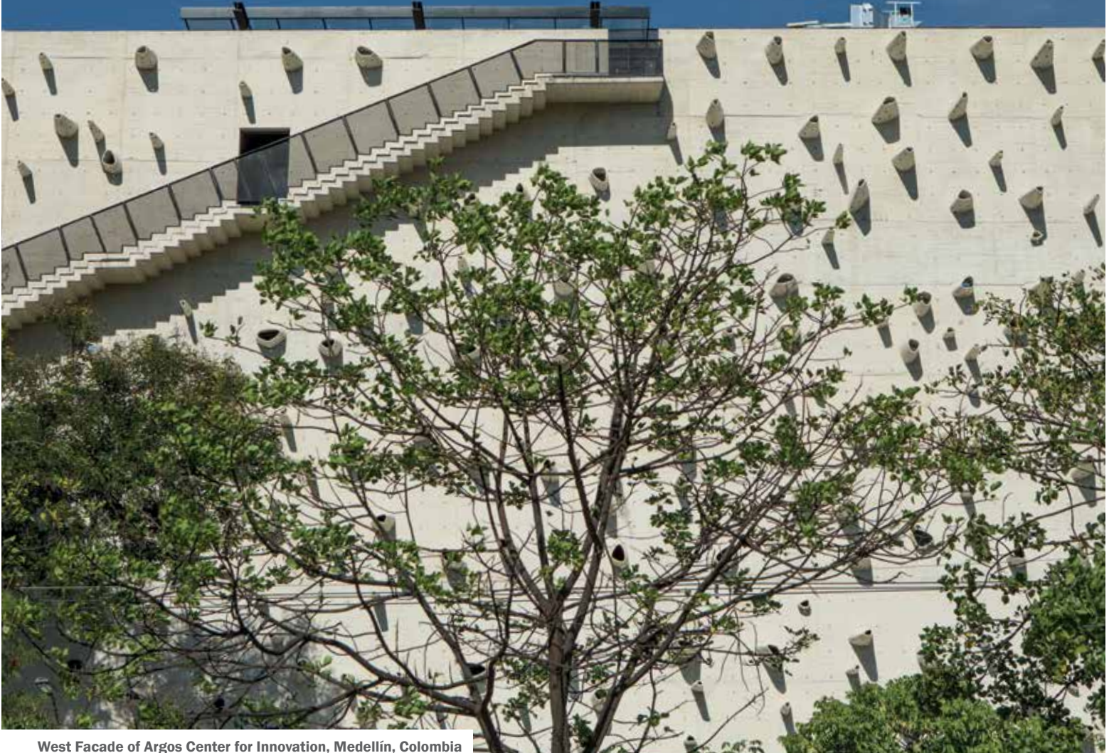
West Facade of Argos Center for Innovation, Medellín, Colombia
