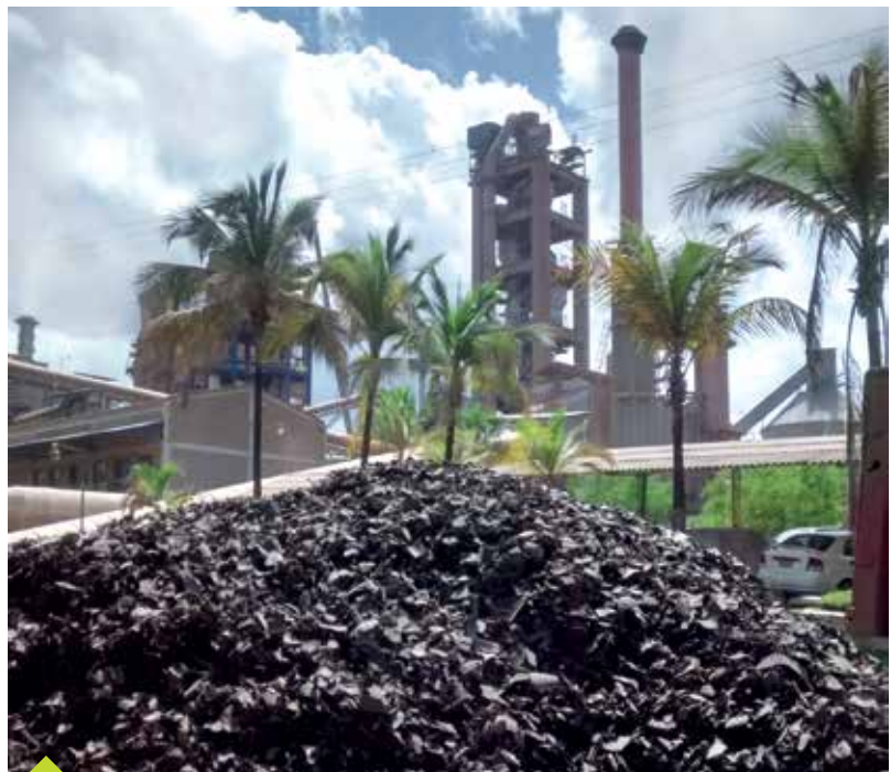
Co-processing at the Rioclaro plant, Colombia Regional Branch
