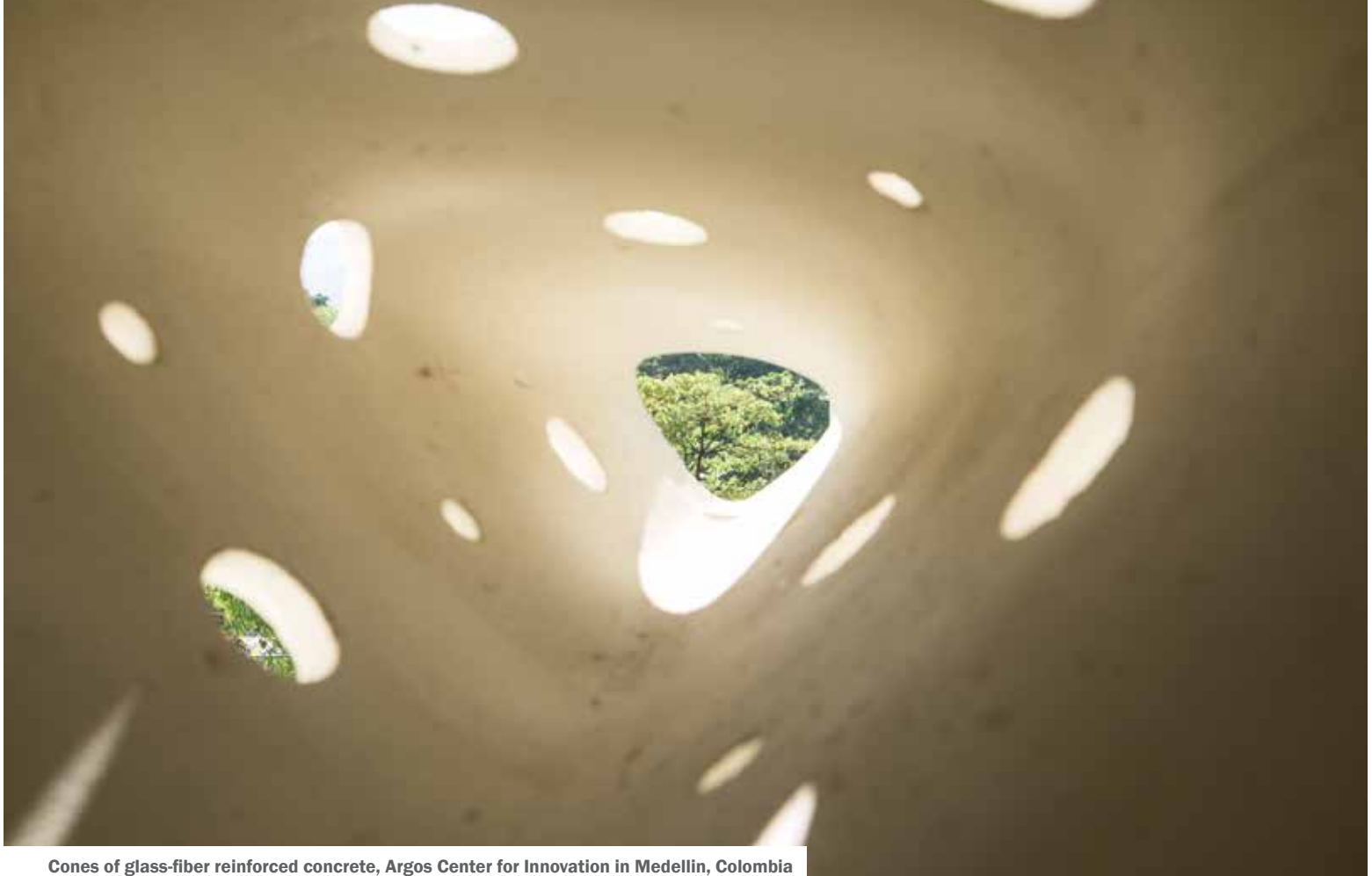
Cones of glass-fiber reinforced concrete, Argos Center for Innovation in Medellin, Colombia
