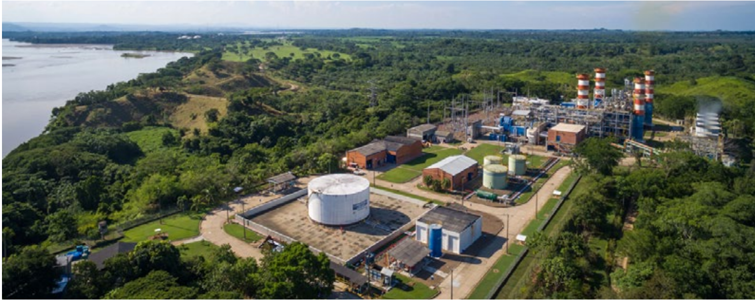
Termocentro Power Plant.
