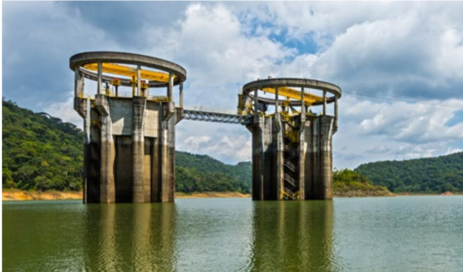
San Carlos Hydroelectric Power Plant
