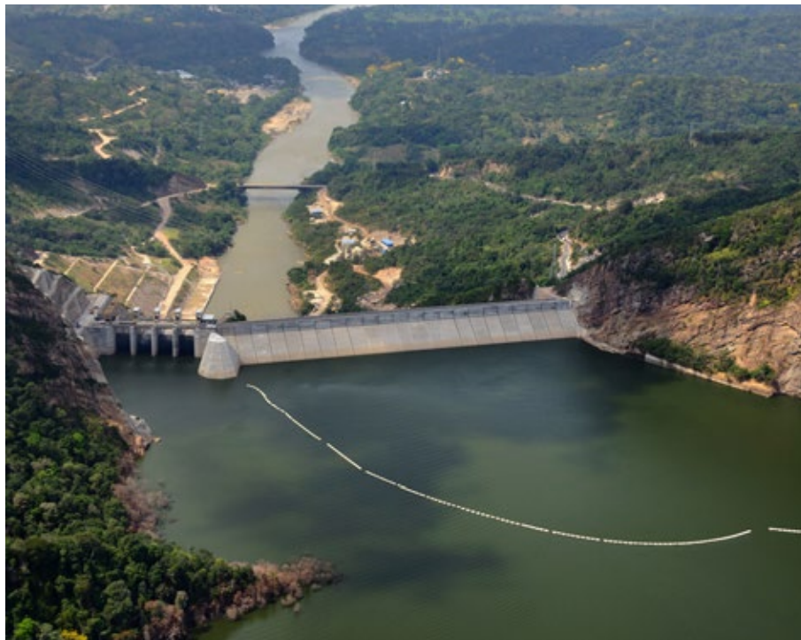
Topocoro Reservoir. Sogamoso Hydroelectric Power Plant.
