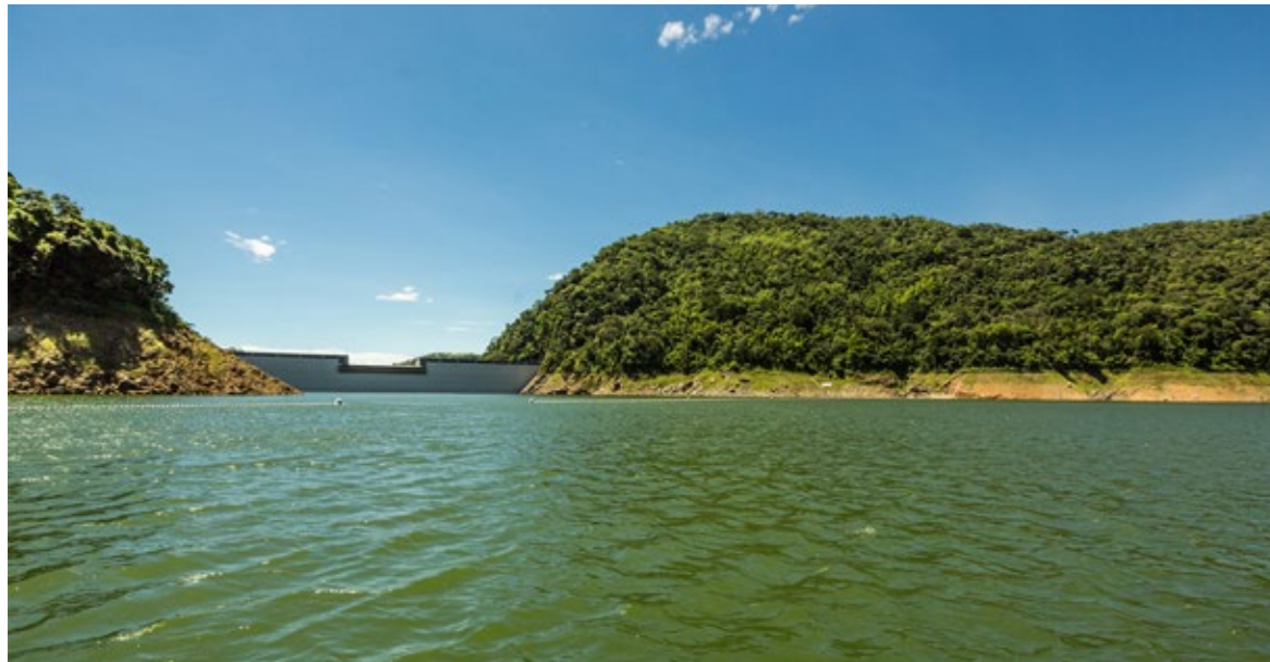
Amaní reservoir. Miel I Hydroelectric Power Plant.
