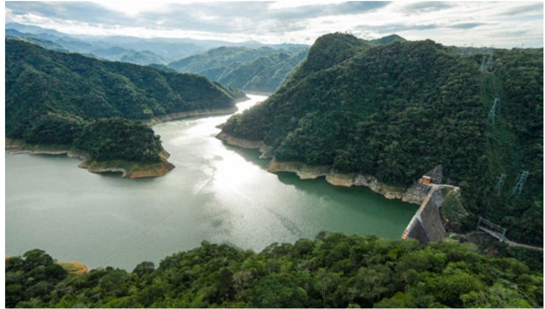
Amaní Reservoir. Miel I Hydroelectric Power Plant.
