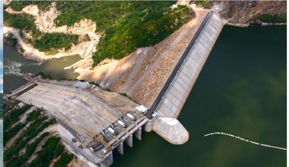
Sogamoso Hydroelectric Power Plant.
