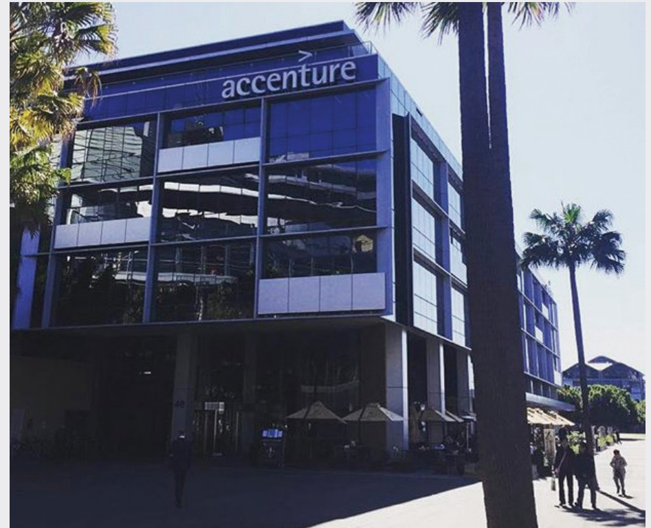
Accenture's office in Sydney is Australia's first building rated 6 Star Green Star, the highest performance rating given by the Green Building Council of Australia.
